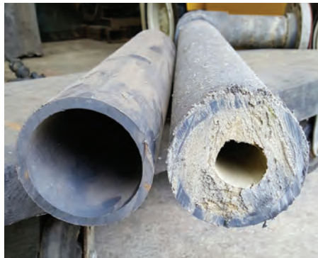
Picture of a 4" line reduced to 1.5" due to grease.
