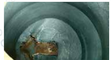
Before and after Sanitary Maintenance Hole Rehab
