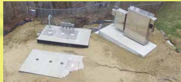
The reconstruction of this major pumping station has been completed and is now in operation. The main structure is 20' below ground where it houses a 7.5 hp pump and 2-35 hp pumps. The waste water travels via a 24" diameter pipe running alongside Route 1 from Cooks Corner to the Sewer District approximately 1.5 miles. This station is designed to constantly feed the treatment plant. This constant feed aids in the overall treatment process as well as savings in electrical costs.
